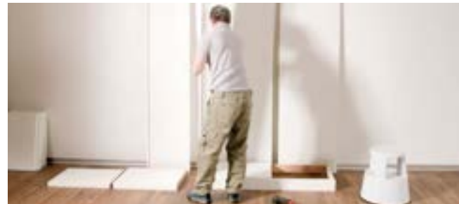
Place furniture side on base. The element is correctly positioned by the protruding screw.
