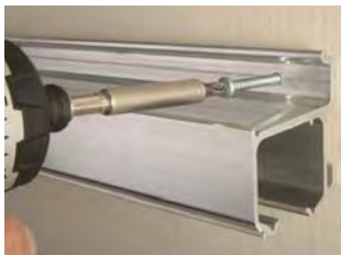
Step 1: Install wall-mount track.
